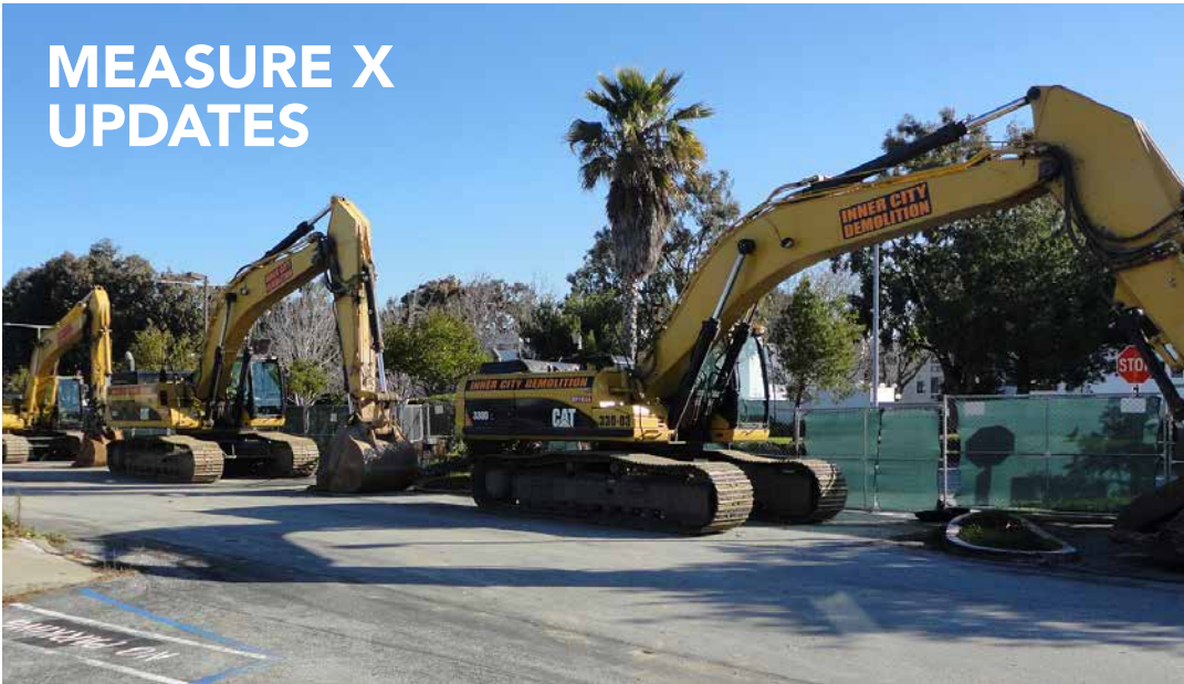
Demolition day at former Charter Square Shopping Center
